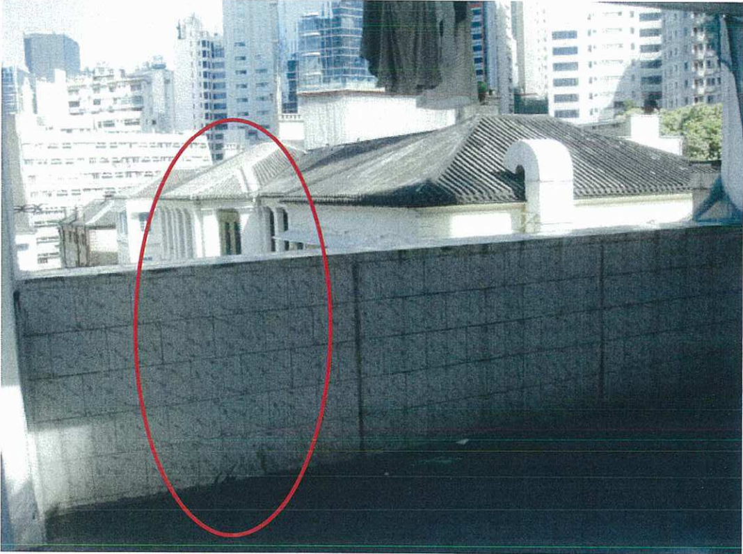
Figure 2 Location of Noise Monitoring Equipment at N2
