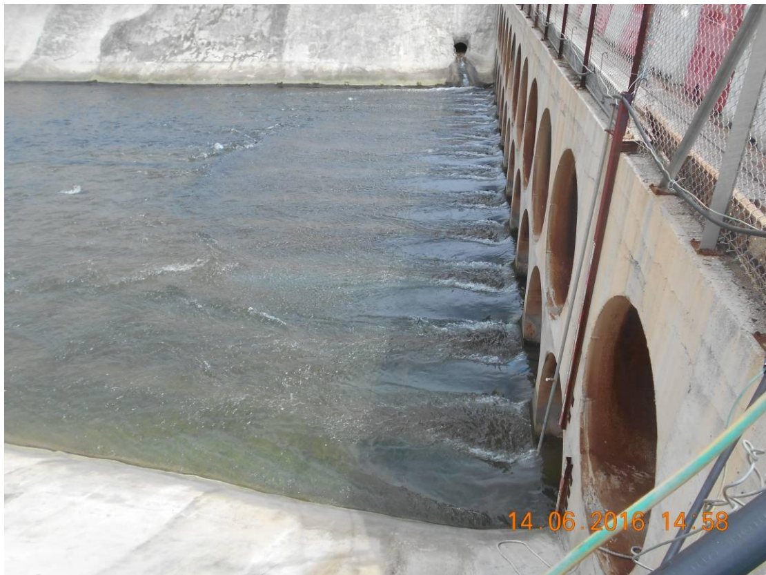
Fig.3–The discharge of site water was treated.
