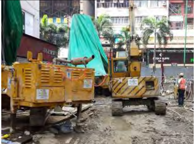
Drill rig located near Nathan Road was fully enclosed by tarpaulin.
