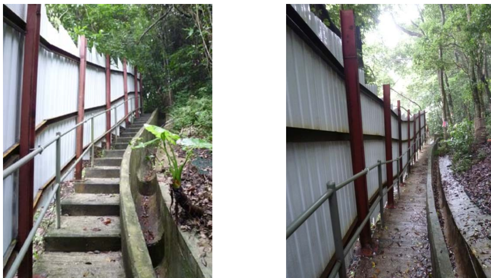
Photo 2 Internal View of Site Hoarding along the Project Boundary
