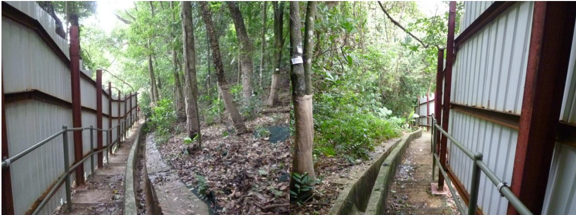
Photo 2 Internal View of Site Hoarding along the Project Boundary
