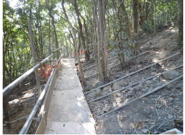
Photo 2 Temporary works area within the project boundary (Section FB1)
