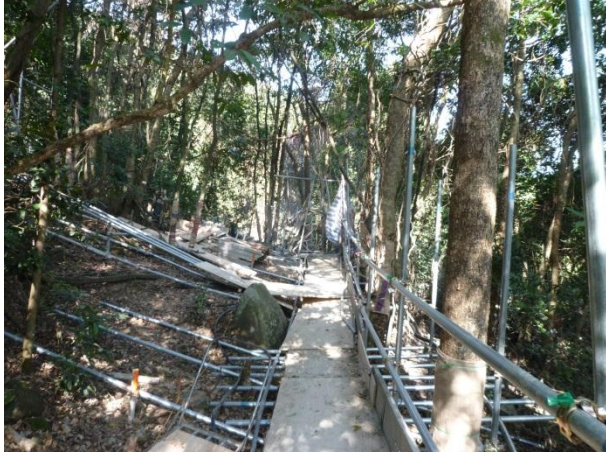
Photo 1 Temporary works area within the project boundary (Section FB1)
