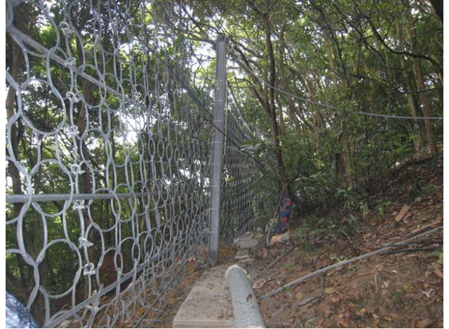
Photo 2 Temporary works area within the project boundary
