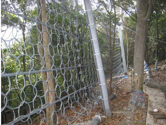
Photo 1 Temporary works area within the project boundary
