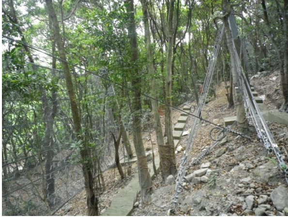
Photo 1 Temporary works area within the project boundary
