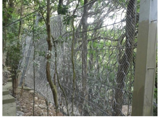
Photo 2 Temporary works area within the project boundary
