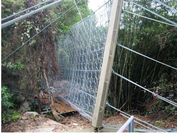
Photo 1 Temporary works area within the project boundary
