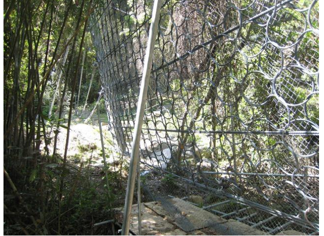
Photo 2 Temporary works area within the project boundary
