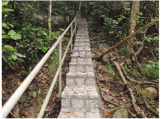
Photo 6 Completed maintenance access
