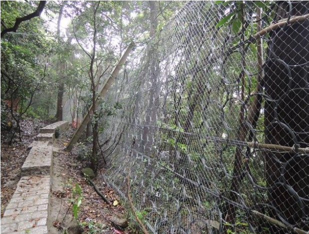
Photo 3 Completed flexible barrier
