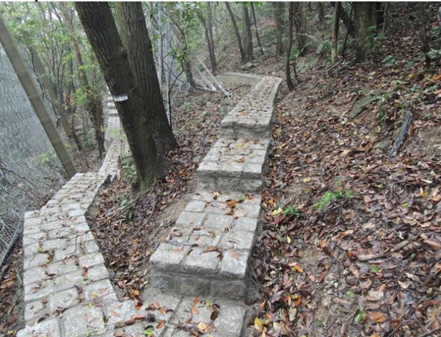
Photo 5 Completed maintenance access
