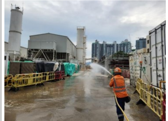
Photo 6 – Watering on the main haul road
