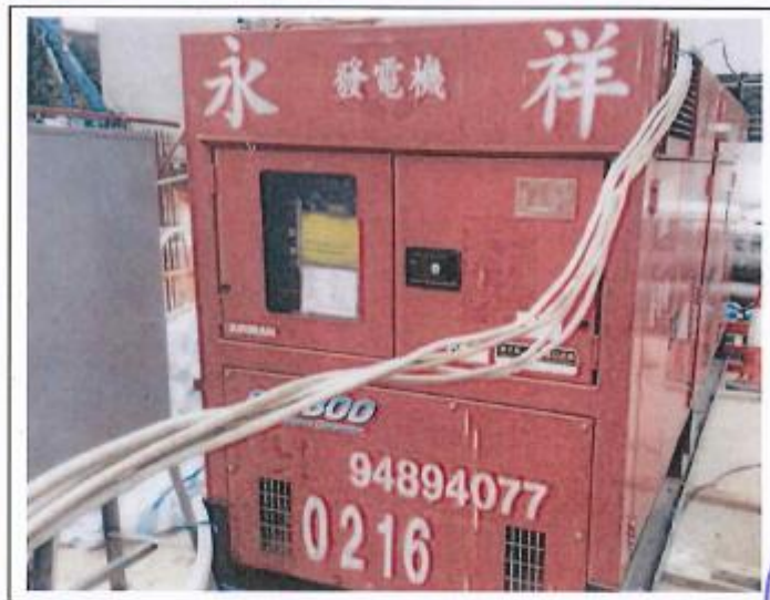
Generator, with Quality Powered Mechanical Equipment Label showing the Sound Power Level of \leq 99 dB(A) 發電機，備有優質機動設備標籤顯示聲功率級 \leq 99 分貝(A)
