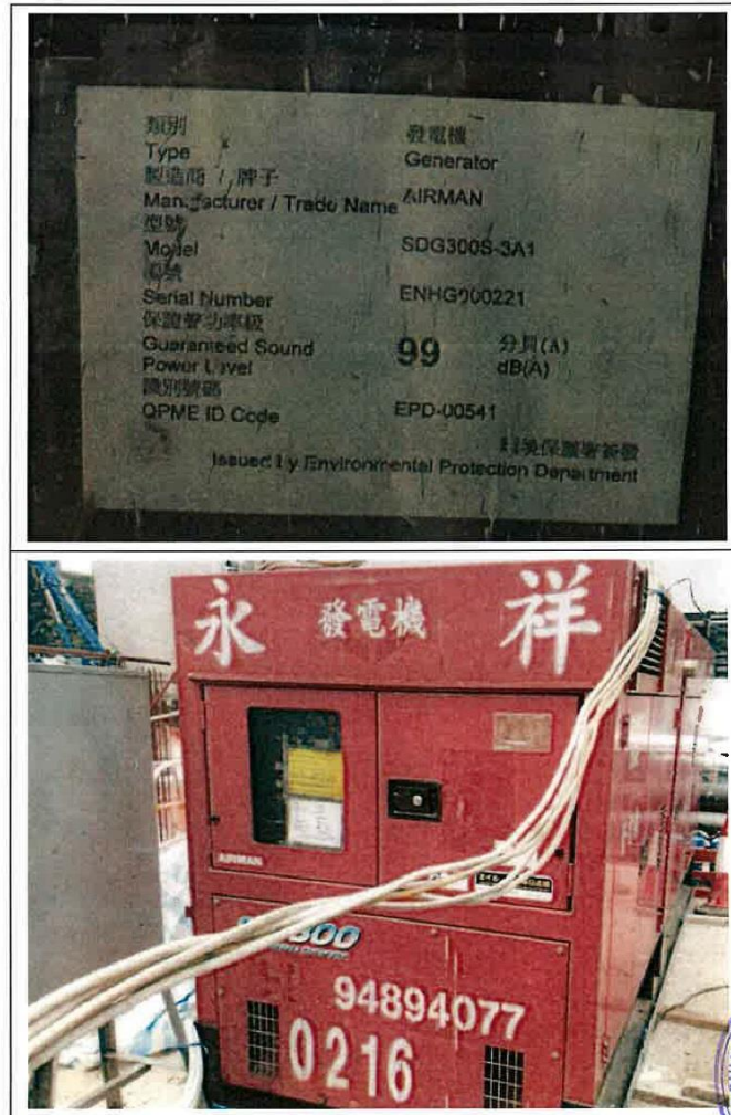
Generator, with Quality Powered Mechanical Equipment Label showing the Sound Power Level of \leq 99 dB(A)
