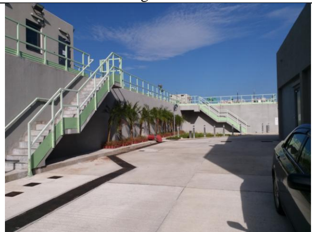
Planting works- groundcovers and potted plants in front of the structure
