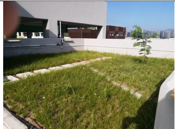
Planting works at roof garden (UV) Figure 10
