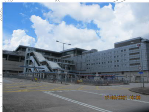
PHOTO 7366: LOK MA CHAU STATION (PHOTO TAKEN: 17 MAY 2021)
