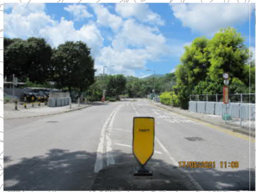
PHOTO 7402: LOK MA CHAU ROAD (PHOTO TAKEN: 17 MAY 2021)
