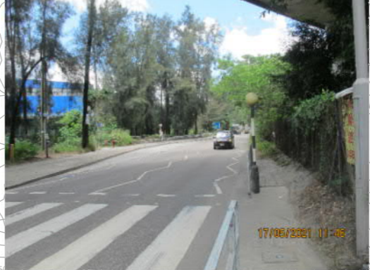
PHOTO 7442: KWU TUNG ROAD (PHOTO TAKEN: 17 MAY 2021)
