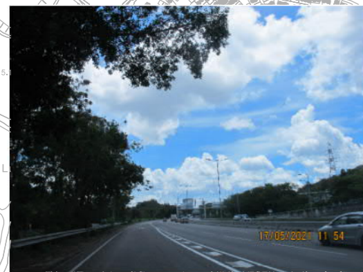
PHOTO 7450: FANLING HIGHWAY (PHOTO TAKEN: 17 MAY 2021)
