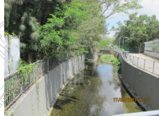
PHOTO 7432: NULLAH (PHOTO TAKEN: 17 MAY 2021)
