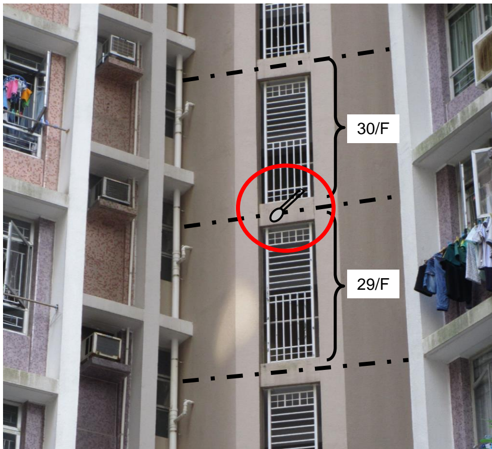
Figure 4 Indicative photo of equipment set up viewing from outside of the building
