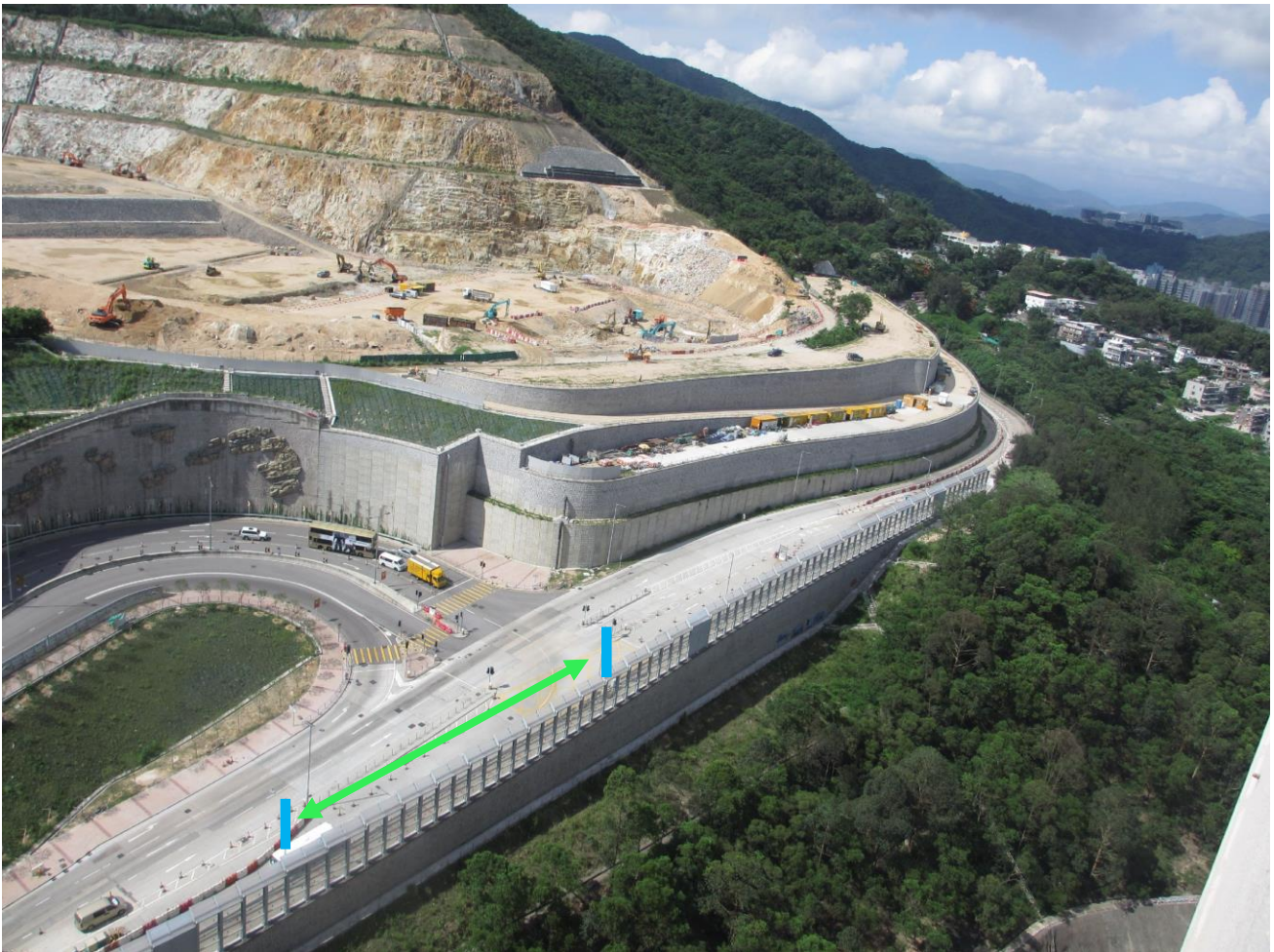
Figure 6 Location of measuring speed of vehicle on west bound of Po Lam Road at Tat Chui House rooftop
