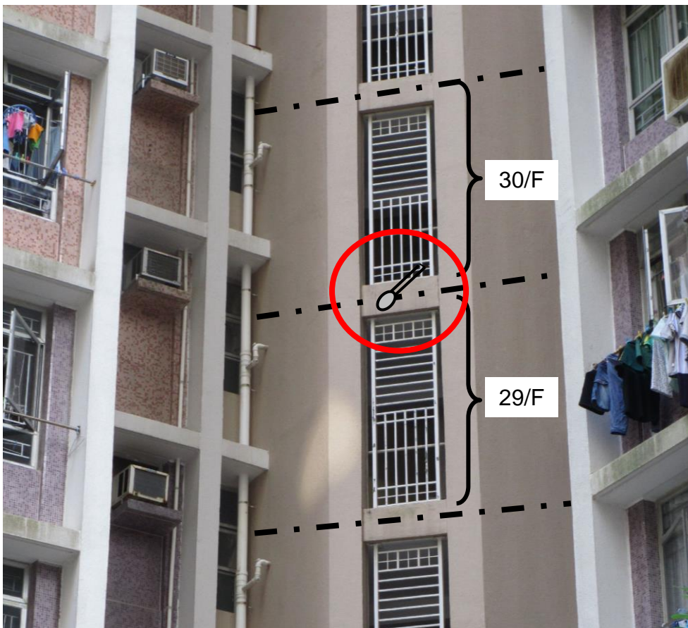
Figure 4 Indicative photo of equipment set up viewing from outside of the building
