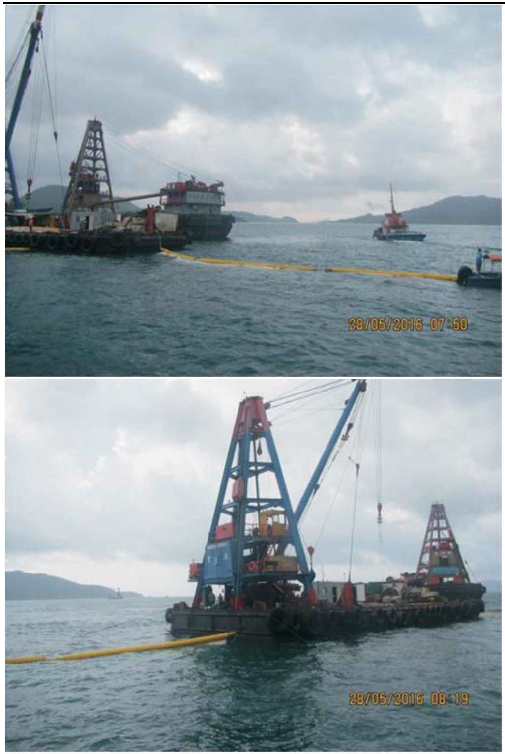
Figure 4.1 Photos of the Installed Silt Curtains for the Project (See Yellow Lines)
