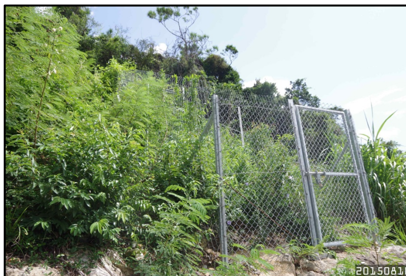
Photo 3 – Temporary Protective Fencing
