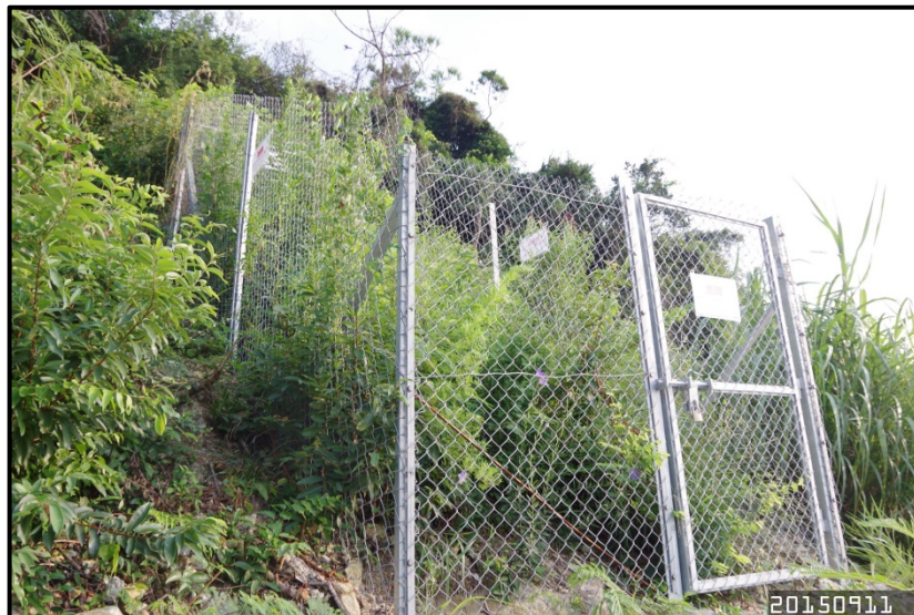
Photo 3 – Currently Situation of Protective Fencing
