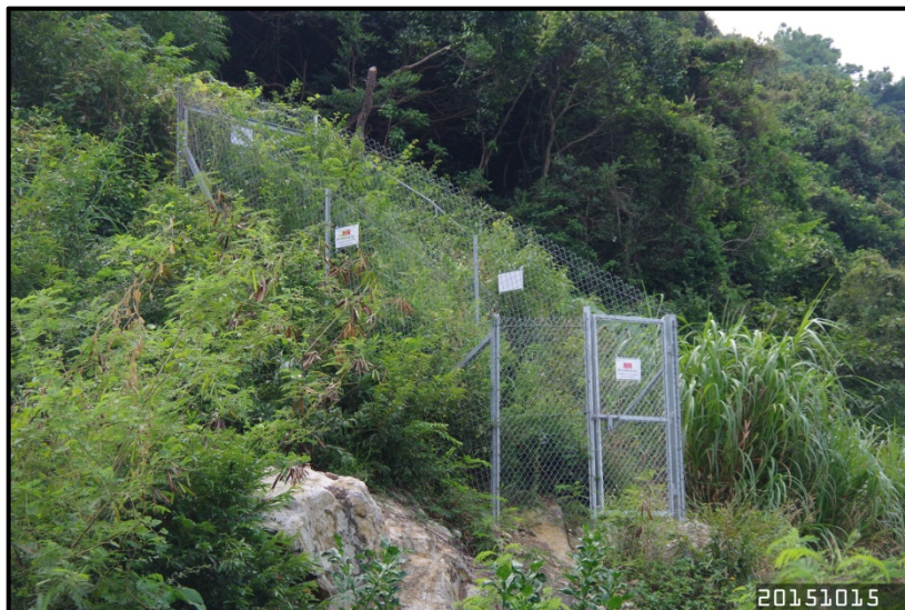
Photo 3 – Currently Situation of Protective Fencing
