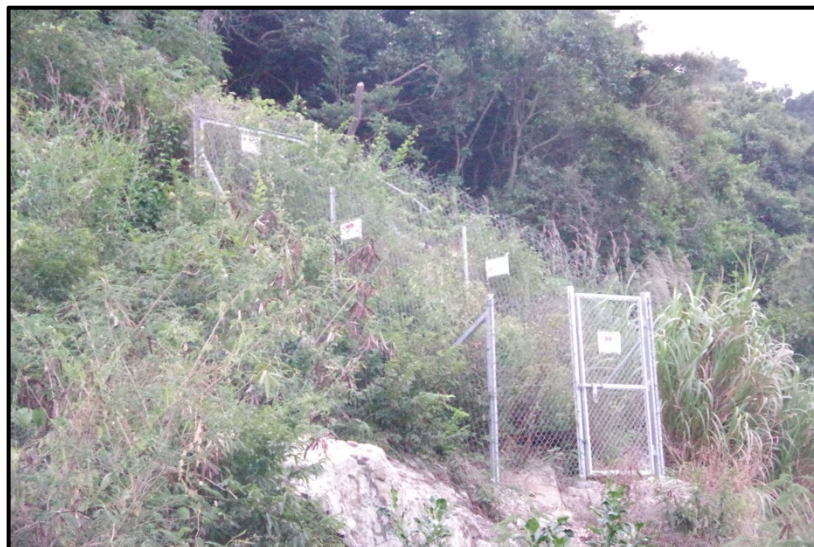
Photo 3 – Currently Situation of Protective Fencing
