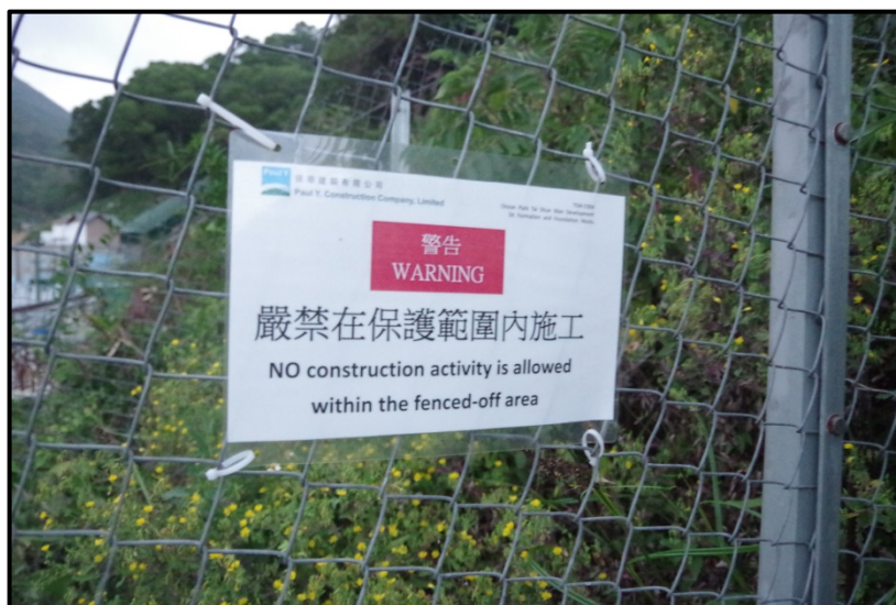
Photo 4 – Warning Sign of Protective Fencing
