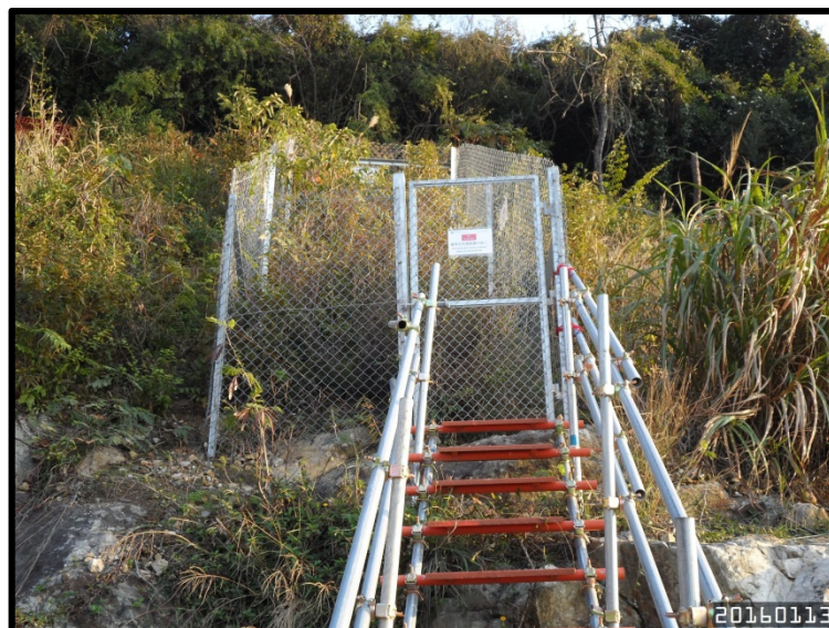
Photo 3 – Currently Situation of Protective Fencing and Warning Sign
