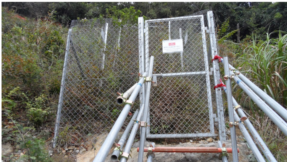
Photo 3 – Currently Situation of Protective Fencing and Warning Sign
