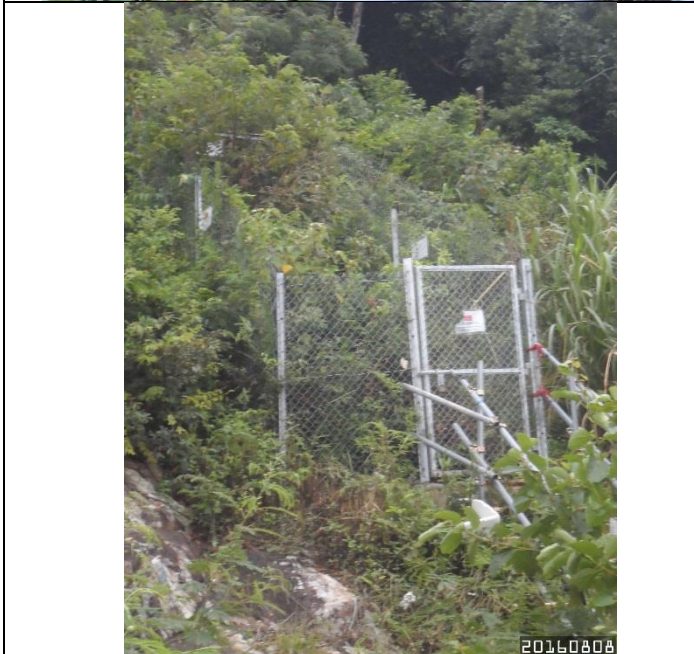
Photo 3 – Currently Situation of Protective Fencing and Warning Sign
