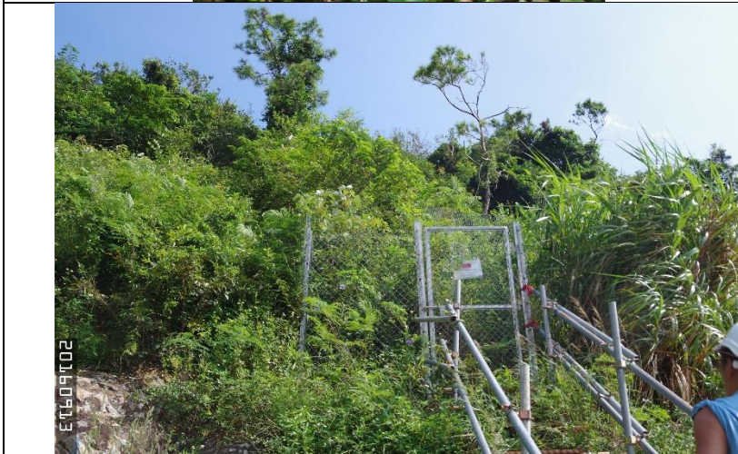
Photo 3 – Currently Situation of Protective Fencing and Warning Sign
