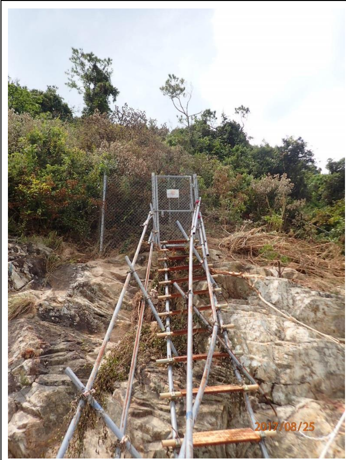
Photo 3 – Current situation of fencing and warning sign
