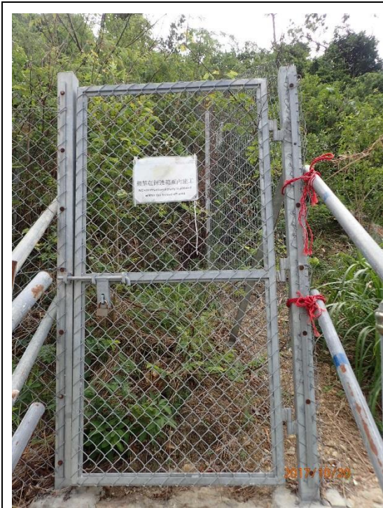
Photo 3 – Current situation of fencing and warning sign
