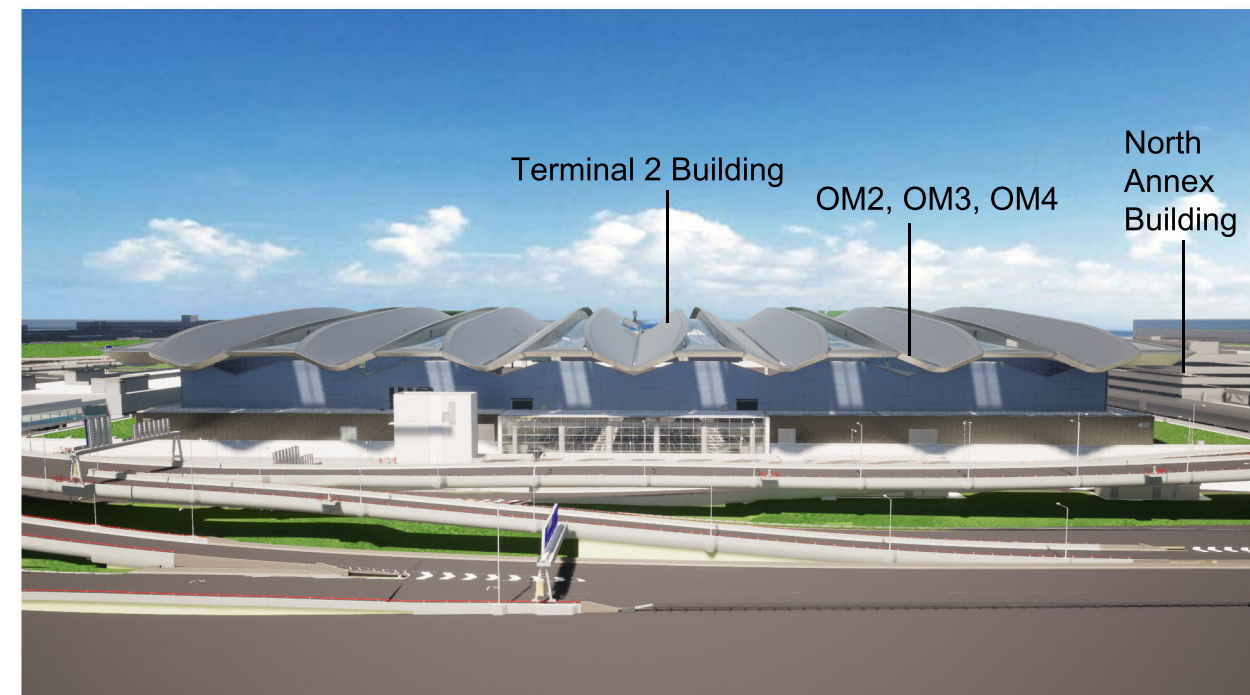
East side of Terminal 2 (T2) Building
