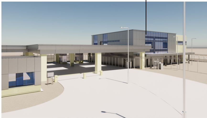
Security Gatehouse View 2
