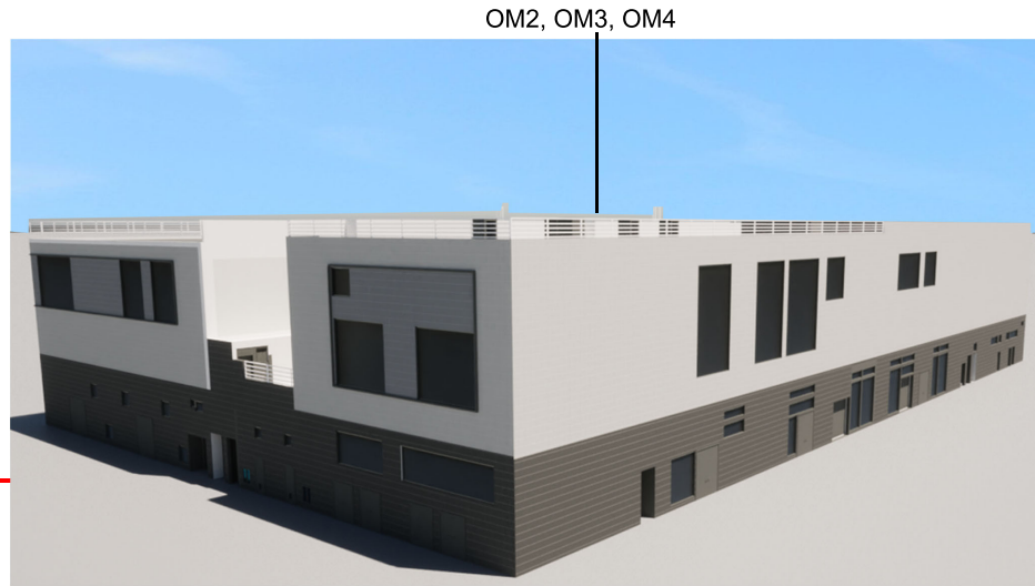
APM BHS Tunnel Vent Building
