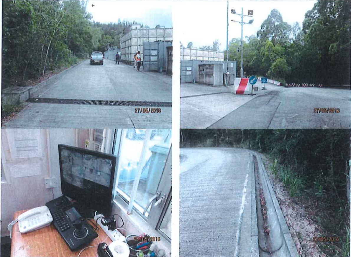
The explosives magazine area is clean and tidy and no environmental issue was observed during the site inspection. (Operation Phase)
