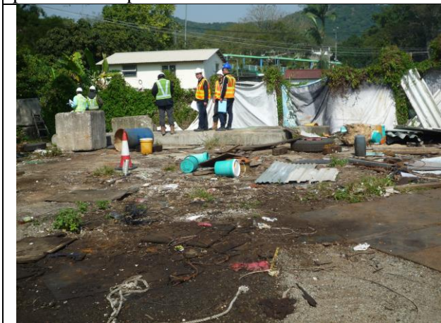
Photo 10 – Oil stain observed at car workshop near entrance.
