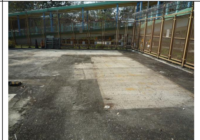
Photo 4 –Open area at the substation
