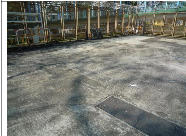
Photo 3 –Open area at the substation
