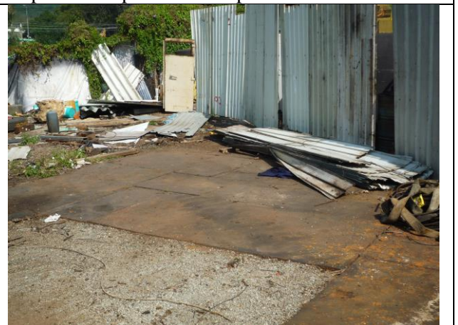
Photo 11 – Material storage on site.
