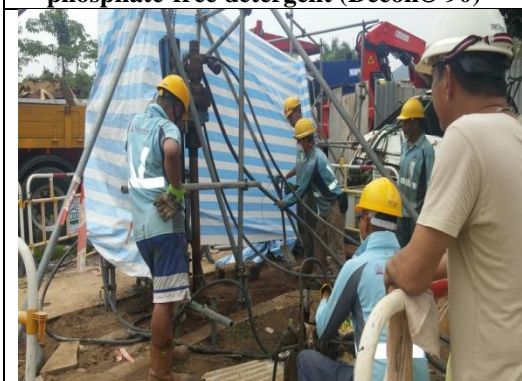
Soil sampling by drilling rig
