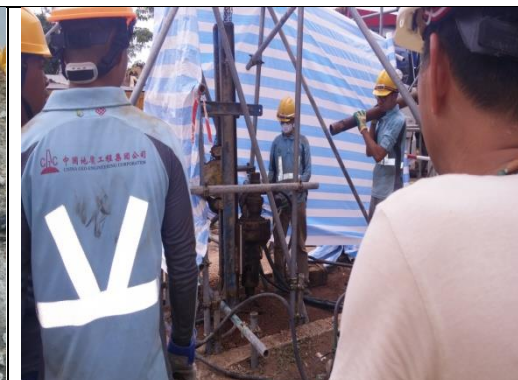
Setting up drilling rig
