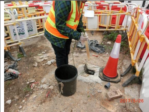
Purging of the Groundwater well
