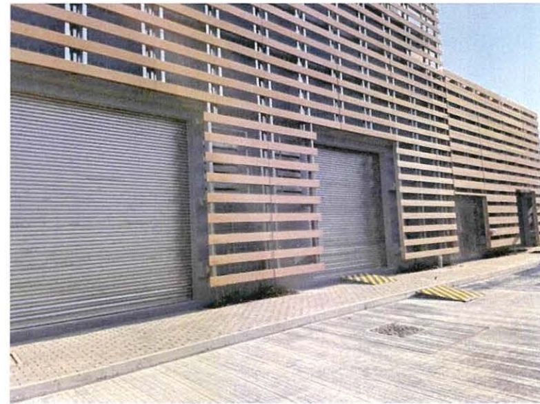
Photo 4 – Roller Shutter and Soundproof Door
