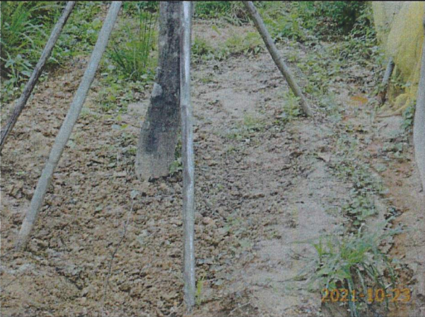
Formation of ditch to guide surface runoff to water pumping location
