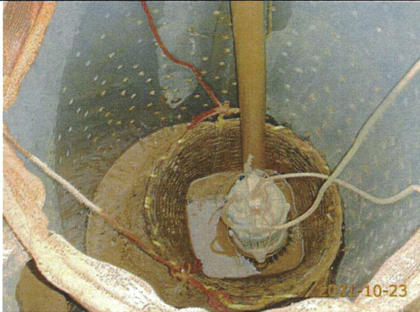
Regular Dewatering at transplanted area
