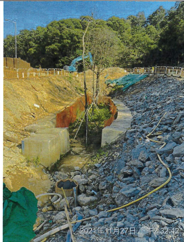
Formation of ditch to guide surface runoff to water pumping location
