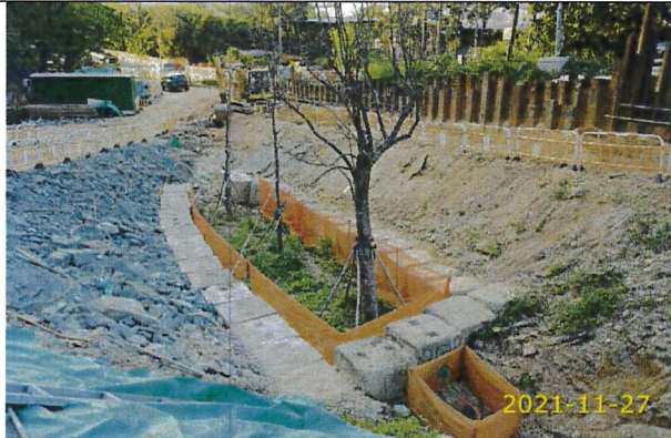
Formation of ditch to guide surface runoff to water pumping location
