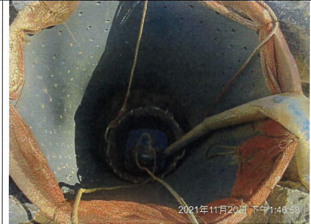
Regular Dewatering at transplanted area
