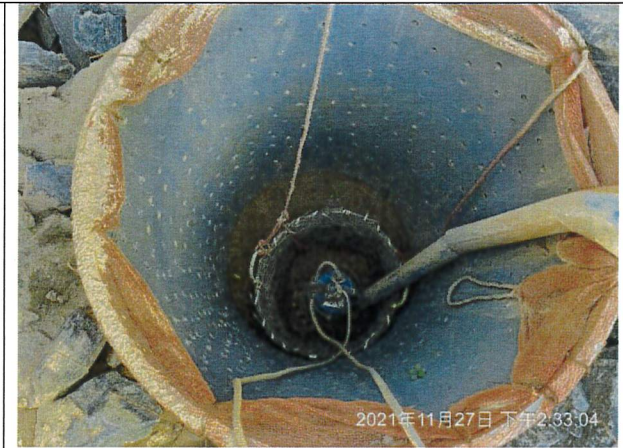
Regular Dewatering at transplanted area
