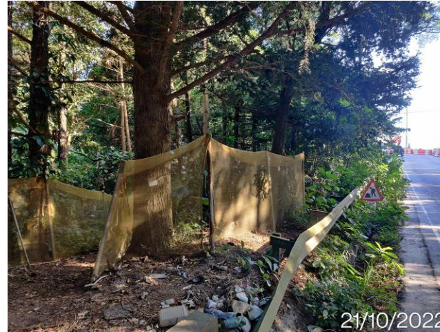
Description: Protective fence for undersized seedling of Aquilaria sinensis are properly erected.
