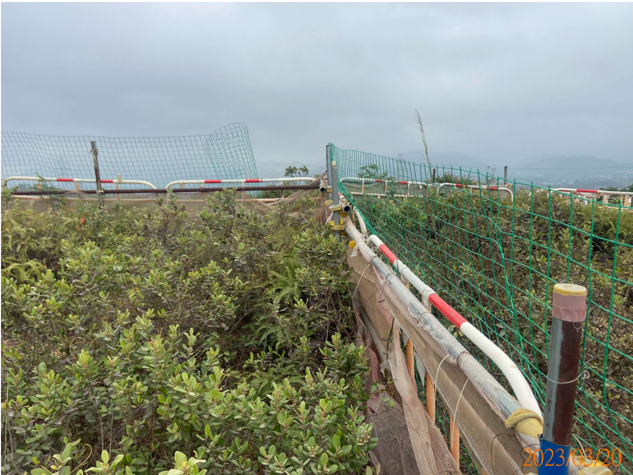
Installation of protection fence (1)
