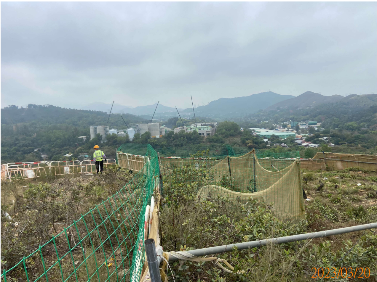
Installation of protection fence (2)
