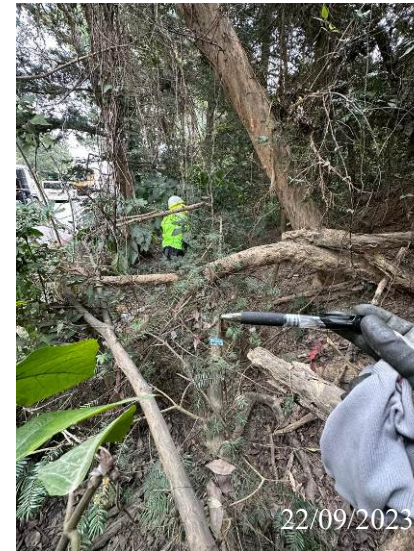
F-0015 was found collapsed in the reporting month after typhoon / adverse weather condition.
