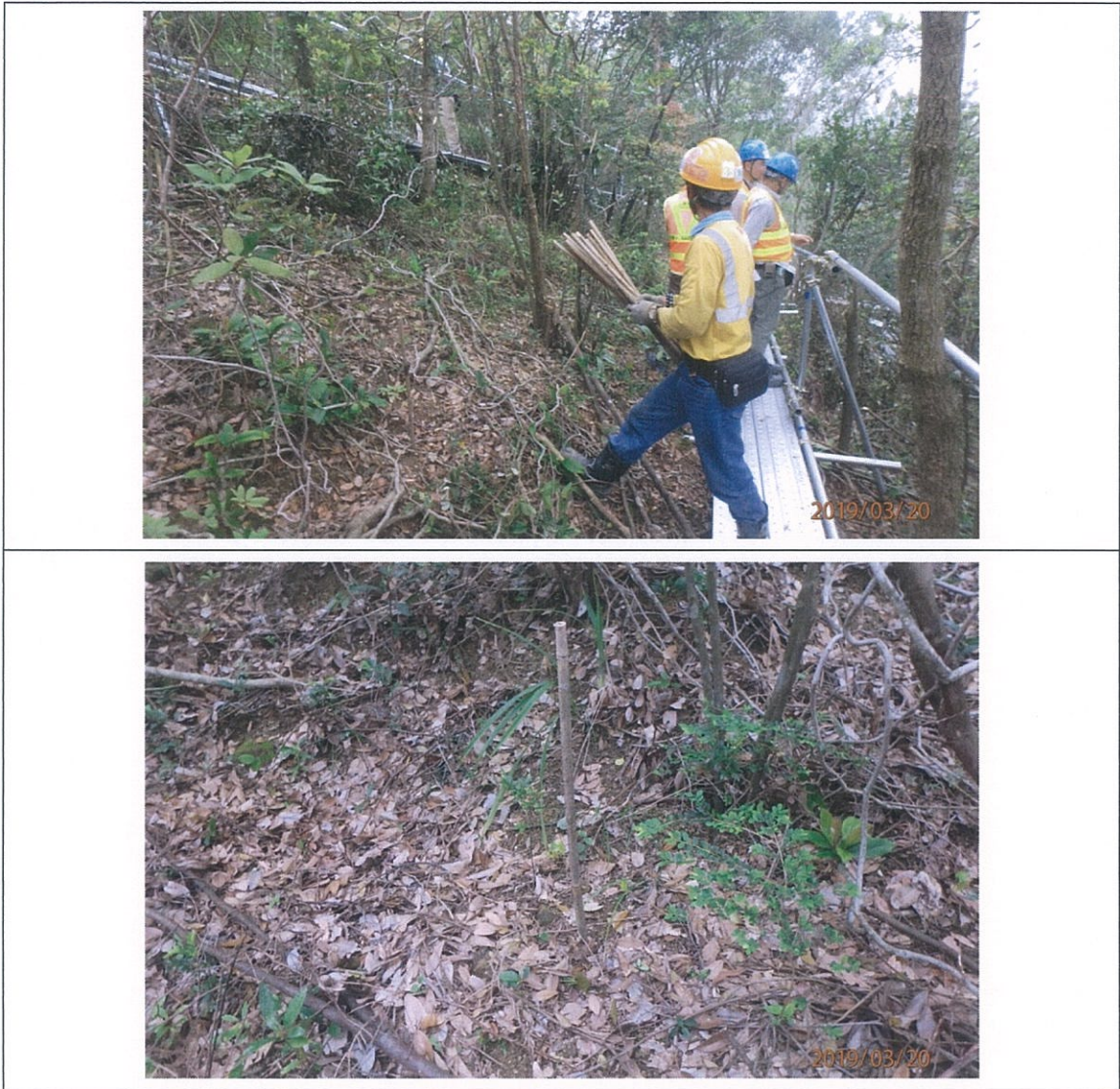
Plate 2. Each planting pit agreed by the Plant Specialist and the Supervisor of the Contract was marked by a bamboo stick prior to transplantation.
