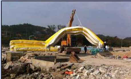
Handling of the silt curtain
