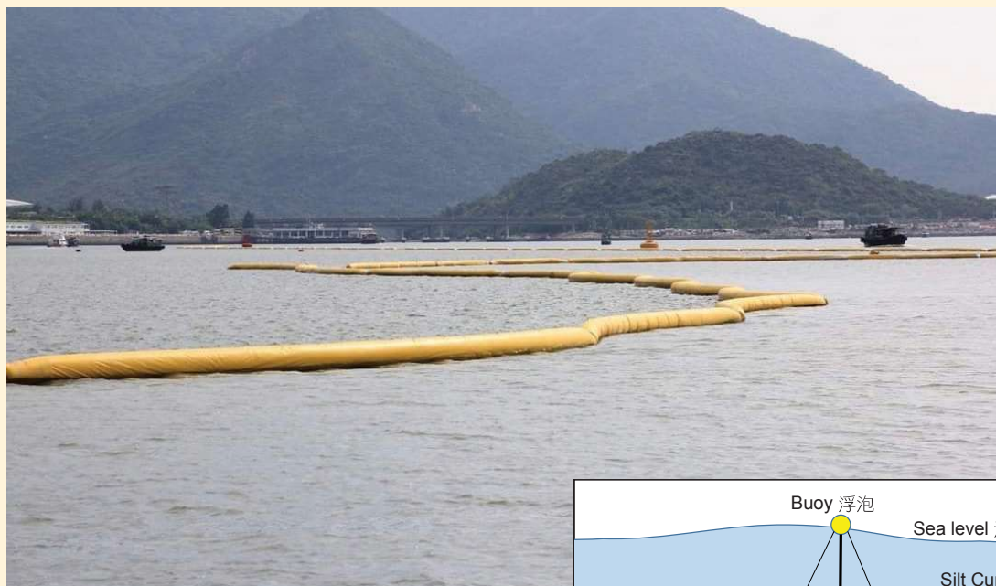
淤泥屏障 Silt curtains
