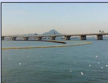
Tung Chung New Town Extension - Reclamation and Advance Works, December 2018 (NL/2017/03)
