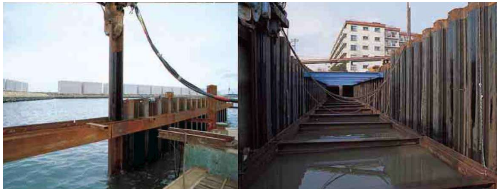
Installation/Extraction of Sheetpile by Vibratory Method
