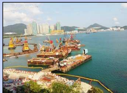
TKO - Lam Tin Tunnel - Main Tunnel and Associated Works, April 2019 (NE/2015/01)
