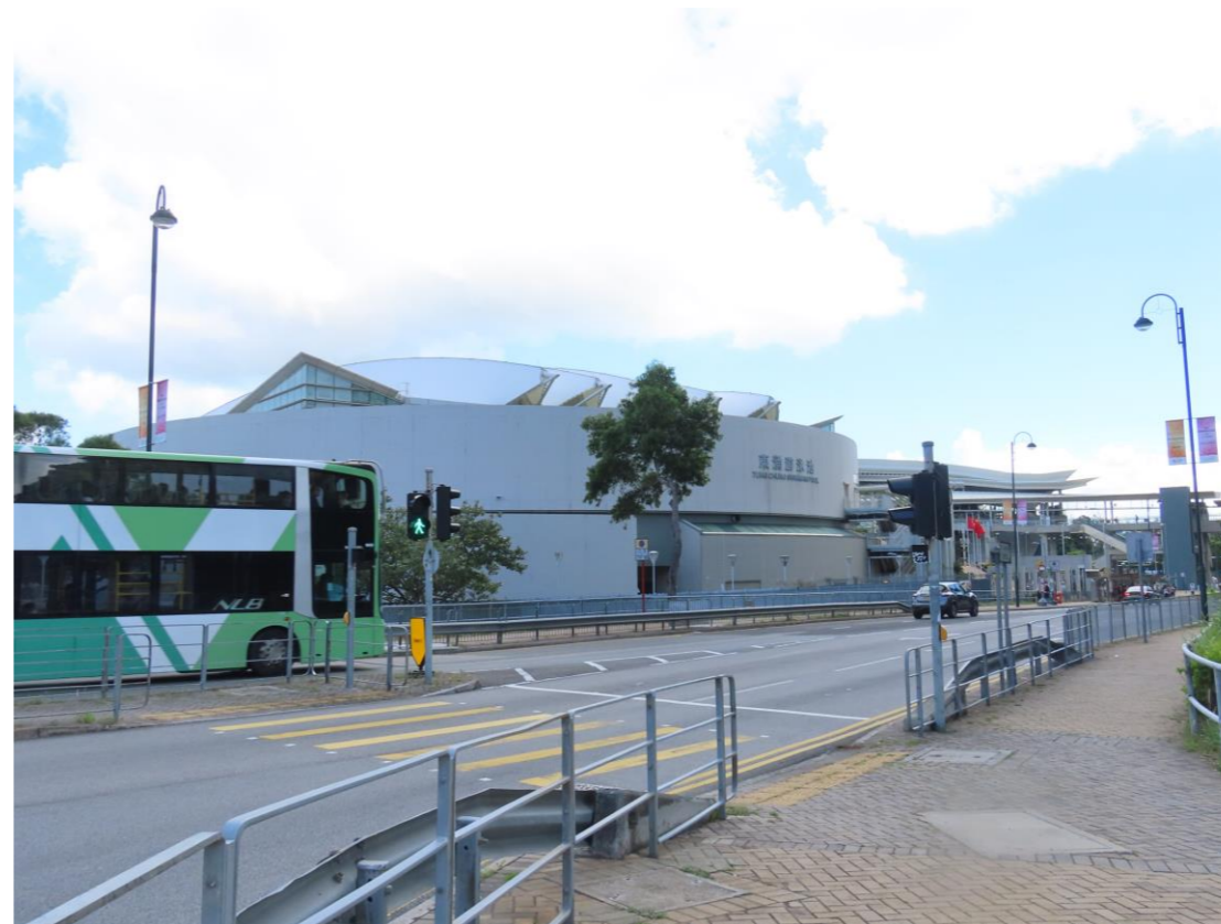
LR 7a Road and Urban Infrastructure
