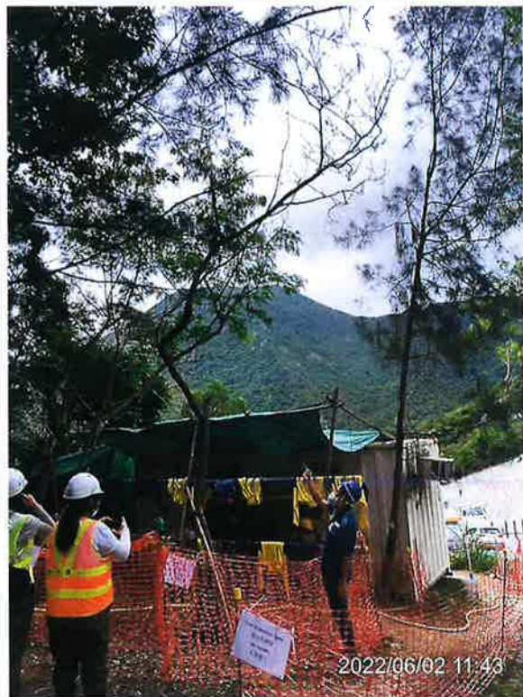
Photo 04: Whole view of G62/RT-07
