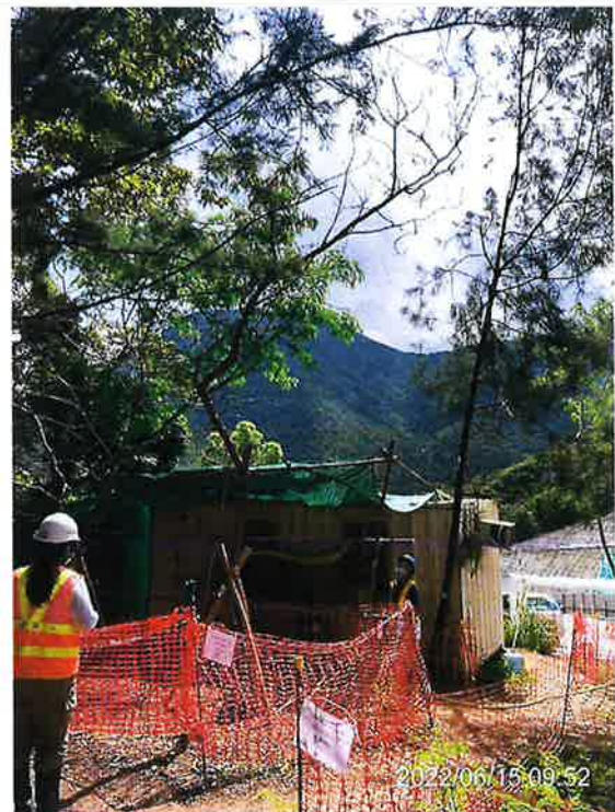
Photo 04: Whole view of G62/RT-07
