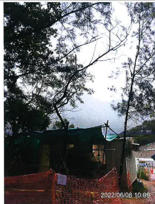
Photo 04: Whole view of G62/RT-07
