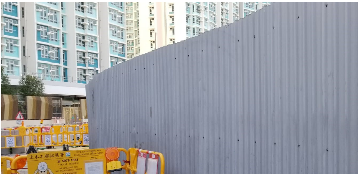
Photo 2 – Erection of site hoardings in unobtrusive colours
