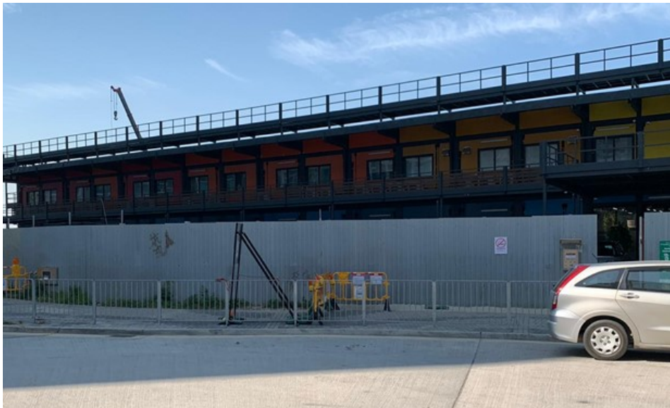
Photo 2 – Erection of site hoardings in unobtrusive colours
