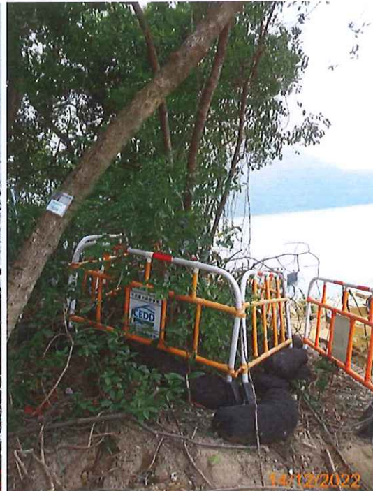
8: Protective fence sealed by sand bag
