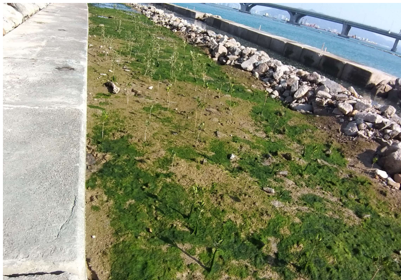
General View of Mangrove Eco-shoreline
