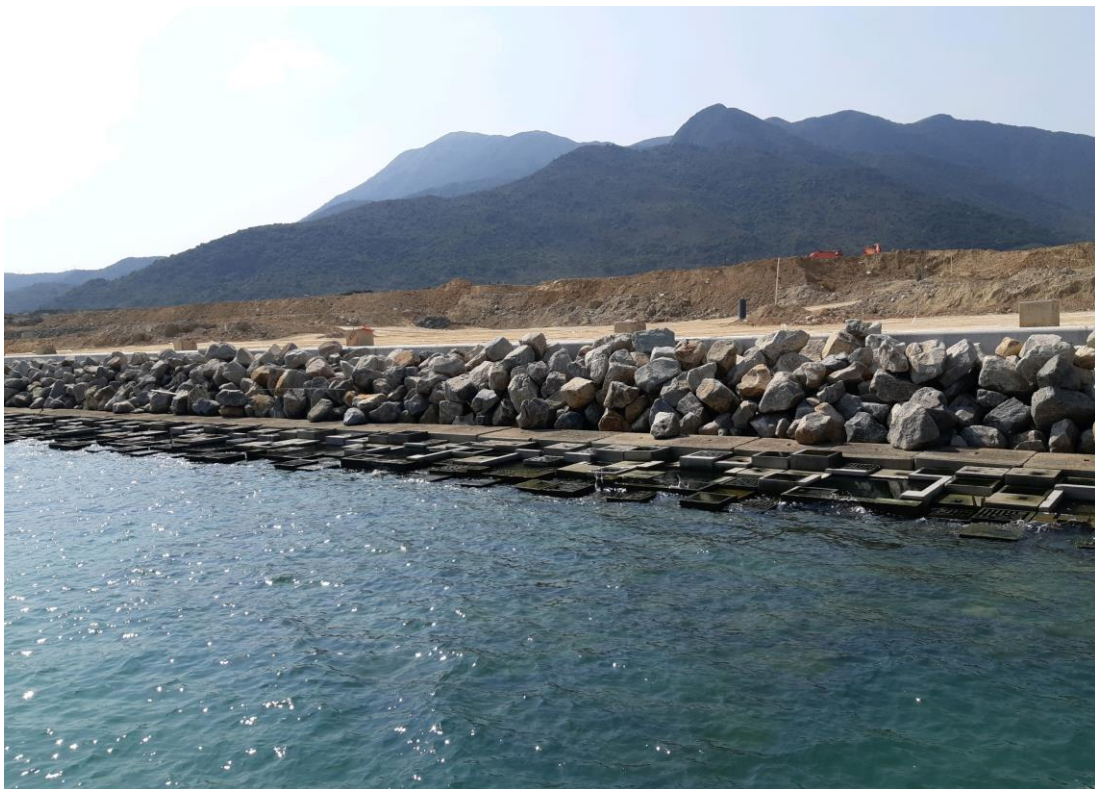
Photo 4 - Natural Rock Material/Planting for Artificial Seawall
