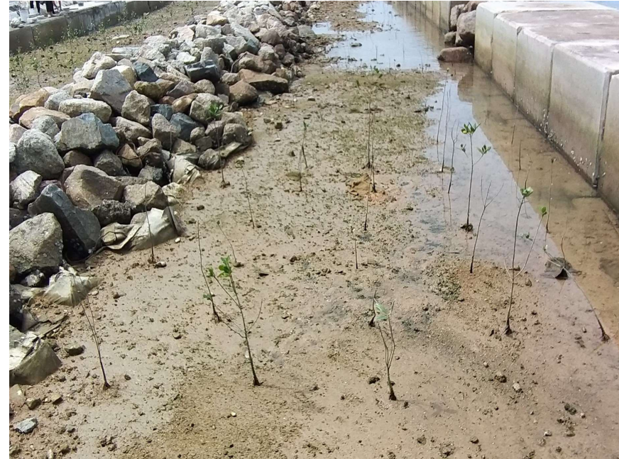
General View of Mangrove Eco-shoreline Lower Terrace
