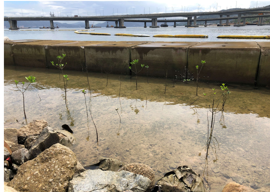
General View of Mangrove Eco-shoreline Lower Terrace
