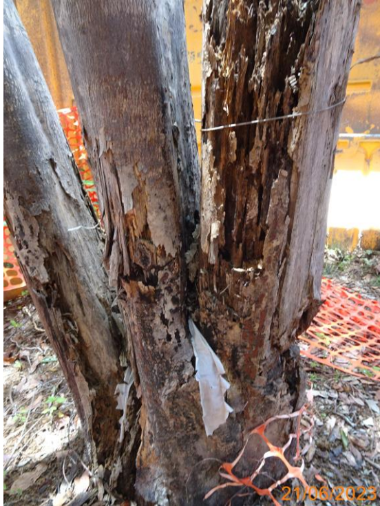
9: U041_ Wood damaged by termite
