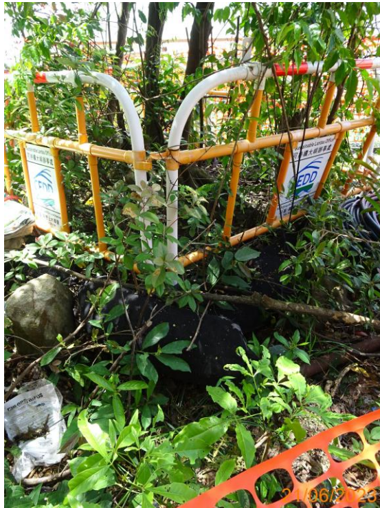
17: Silt rock composed of wood chip was added
