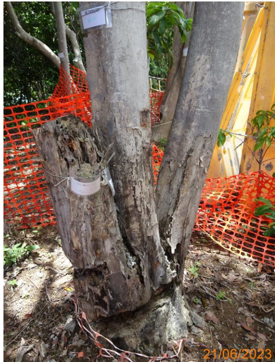
8: U041_Wood damage at union
